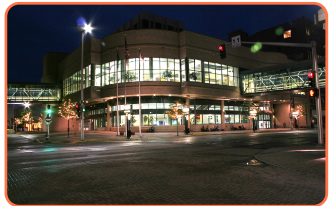
STA Plaza at night
